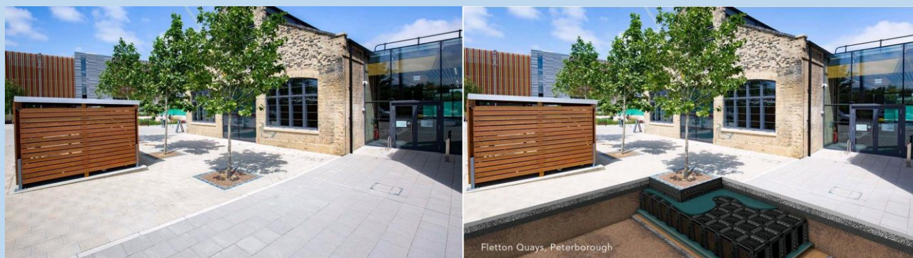
Figure 3-4: Wildlife areas, rain gardens and tree pits were incorporated into Fletton Quays redevelopment (photo provided by GreenBlue Urban)
